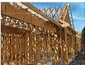
New cottage construction photo by Joy Dryer
